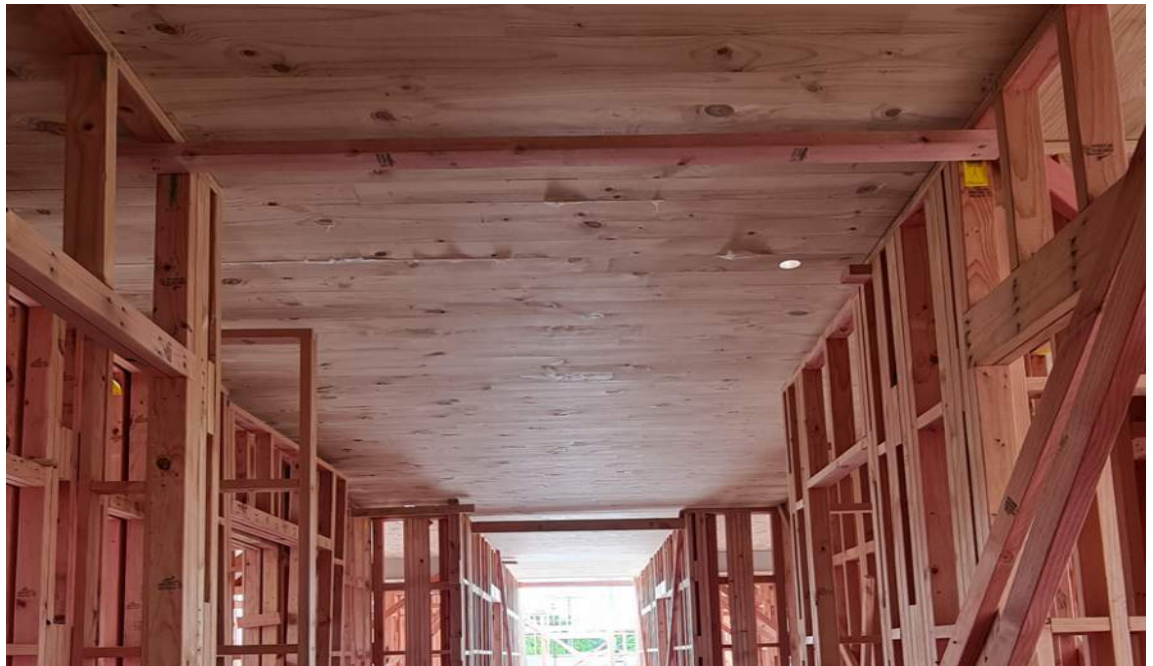
Figure 18: Red Stag CLT midfloor over the Red Stag light timber framing (Red Stag has a frame and truss manufacturing plant in Hamilton, New Zealand that can integrate supply into a hybrid mass and light timber projects).
