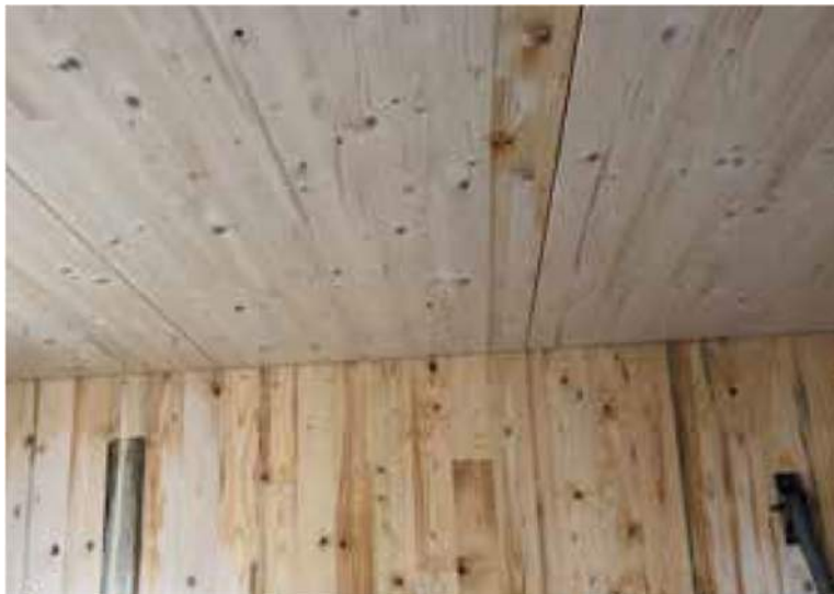
Figure 29: Stains due to water ingress [2] .
