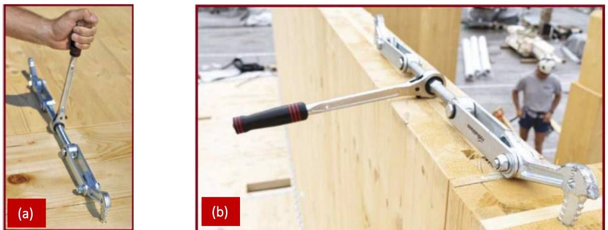
Figure 89: SKORPIO applications; a) SKORPIO utilised to pull CLT floor panels together; b) SKORPIO utilised to pull CLT wall panels together (pulling into a corner) [20] .
