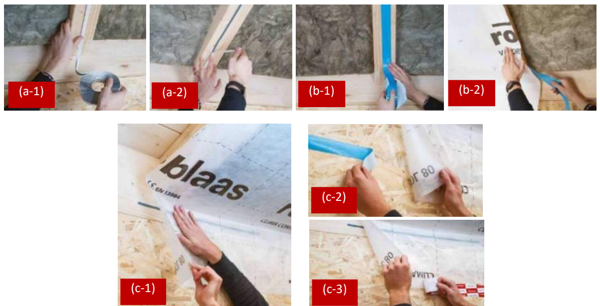
Figure 45: Application on internal side of the roof [14] .
