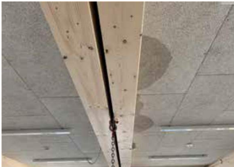
Figure 31: Leaking joint in mass timber [2] .
