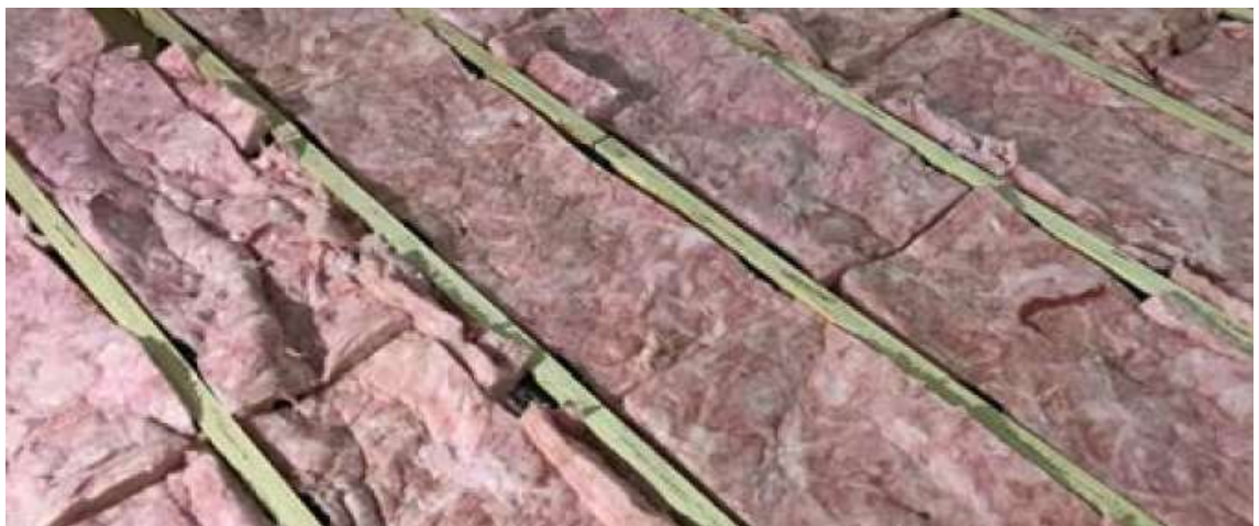
Figure 160: Cradle system with thermal insulation.
