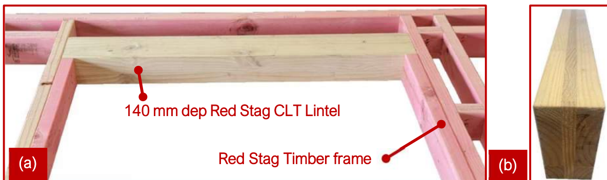
Figure 200: Red Stag CLT lintel in a Red Stag Wood Solutions frame; a) Red Stag CLT lintel over a window opening; b) Example of a common Red Stag CLT lintel.
