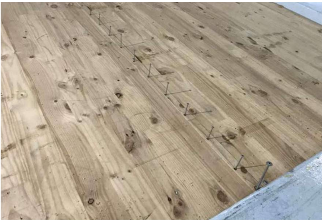
Figure 164: Three-layer Red Stag CLT panel with lap joint.
