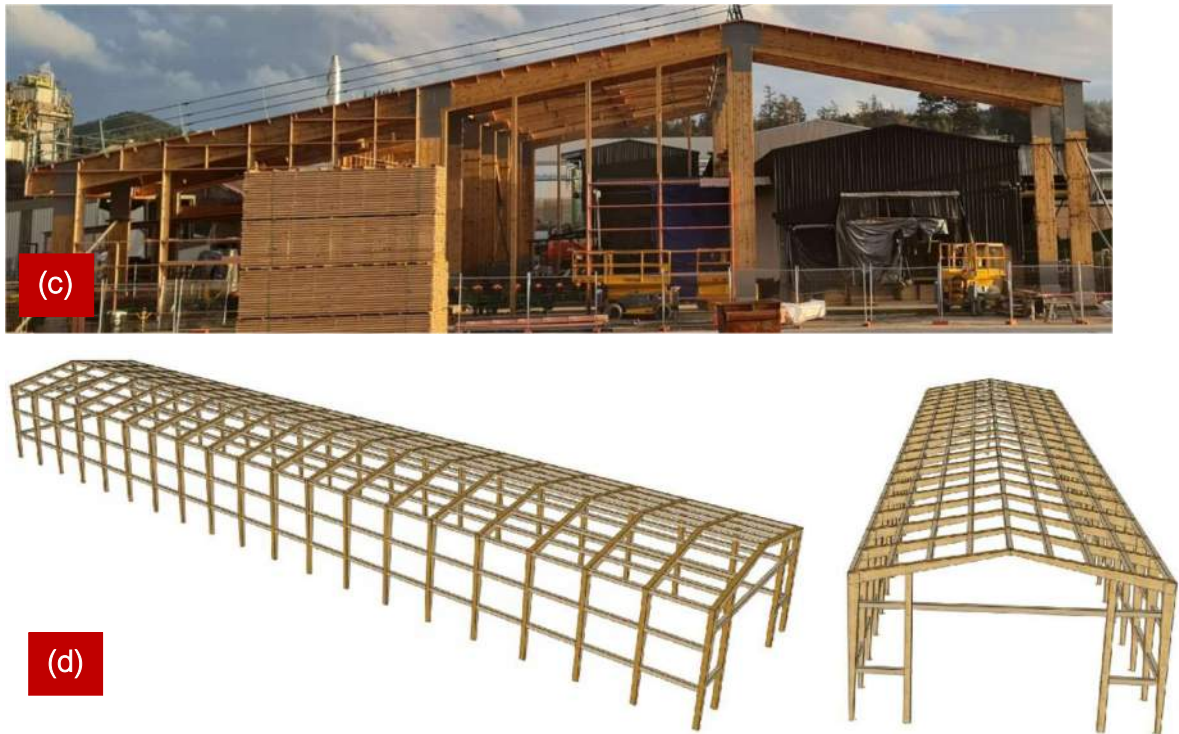
Figure 199: Fast and efficient CNC processing of Red Stag CLT portal frames; a) Optimisation process of CLT portal frame manufacturing; b) Red Stag CNC equipment; c) Parallel CLT portal frame at Red Stag stacker building; d) Truncated CLT Portal frame.
