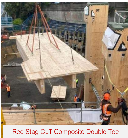
Figure 189: Red Stag CLT composite product installation in Living Pa Project site, Wellington/New Zealand.
