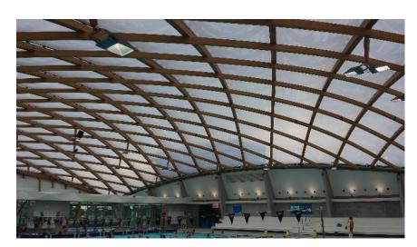
**Cranked Beams** - These beams follow the roof pitch on their top edge while the bottom forms a radius curve. Cranked beams taper from the tangent point to a minimum end depth to provide maximum economy. They may be simply supported on timber or concrete posts.
