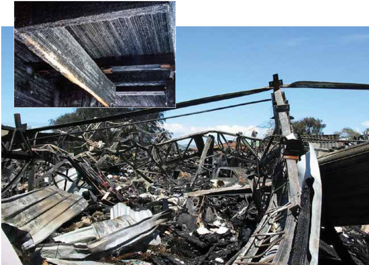
Crown Movers steel portal building post fire. (inset) Glulam floor beams showing significant charring of timber.
