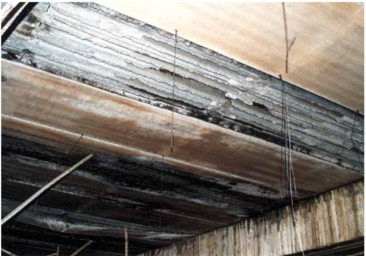
Precast floor panels spalling due to fire.
