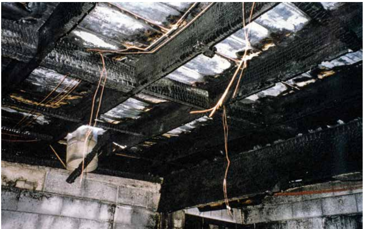
Charred timber roof framing still intact following a fire.
