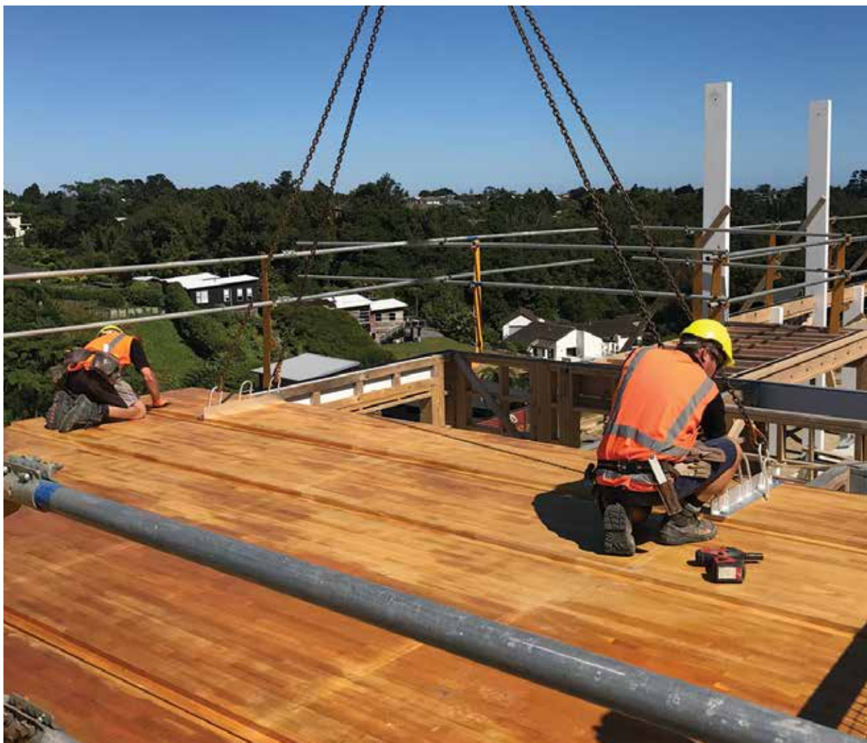
Woodspan PLT Floor being installed. Credit Taranakipine.
