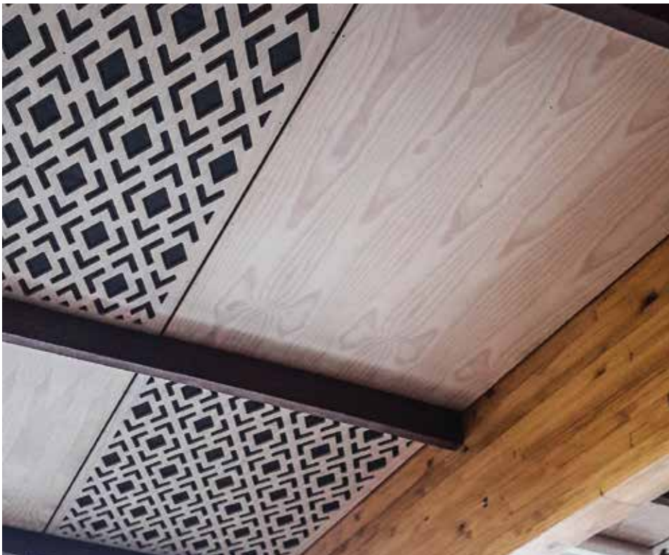
Exposed timber fire rated ceiling (intumescent coating). Credit Resene.
