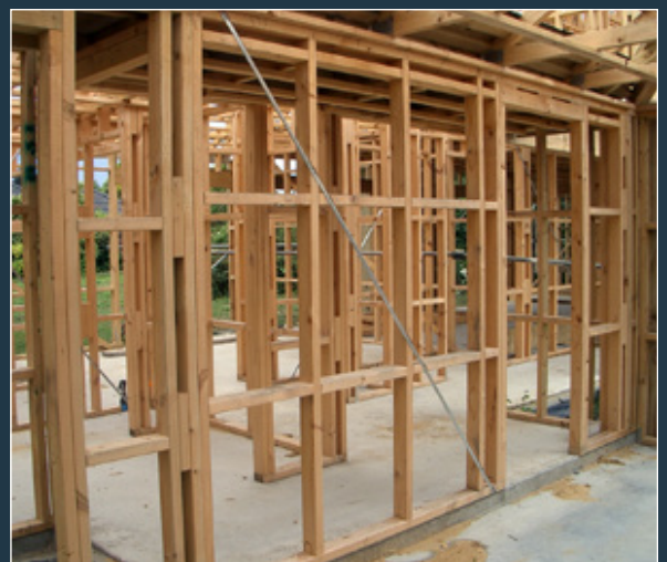
Light steel strap as bracing element in timber housing.
