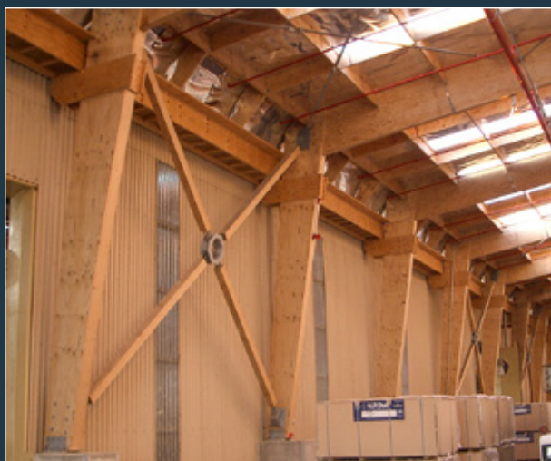
Timber portal frame with timber cross bracing.
