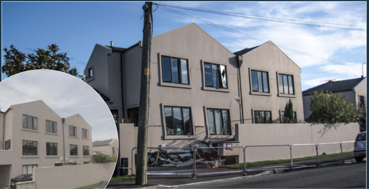
Multi-unit residential housing that suffered a soft-storey collapse during an aftershock of the Christchurch earthquake.
