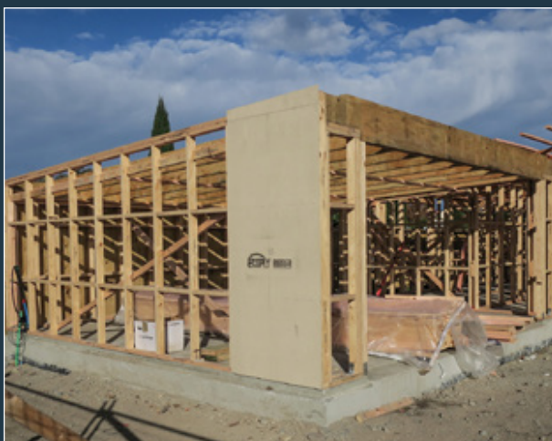
A single storey light timber frame building with a plywood bracing panel.
