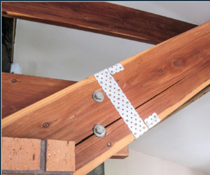
Damage to notched timber member following the Christchurch earthquakes.
