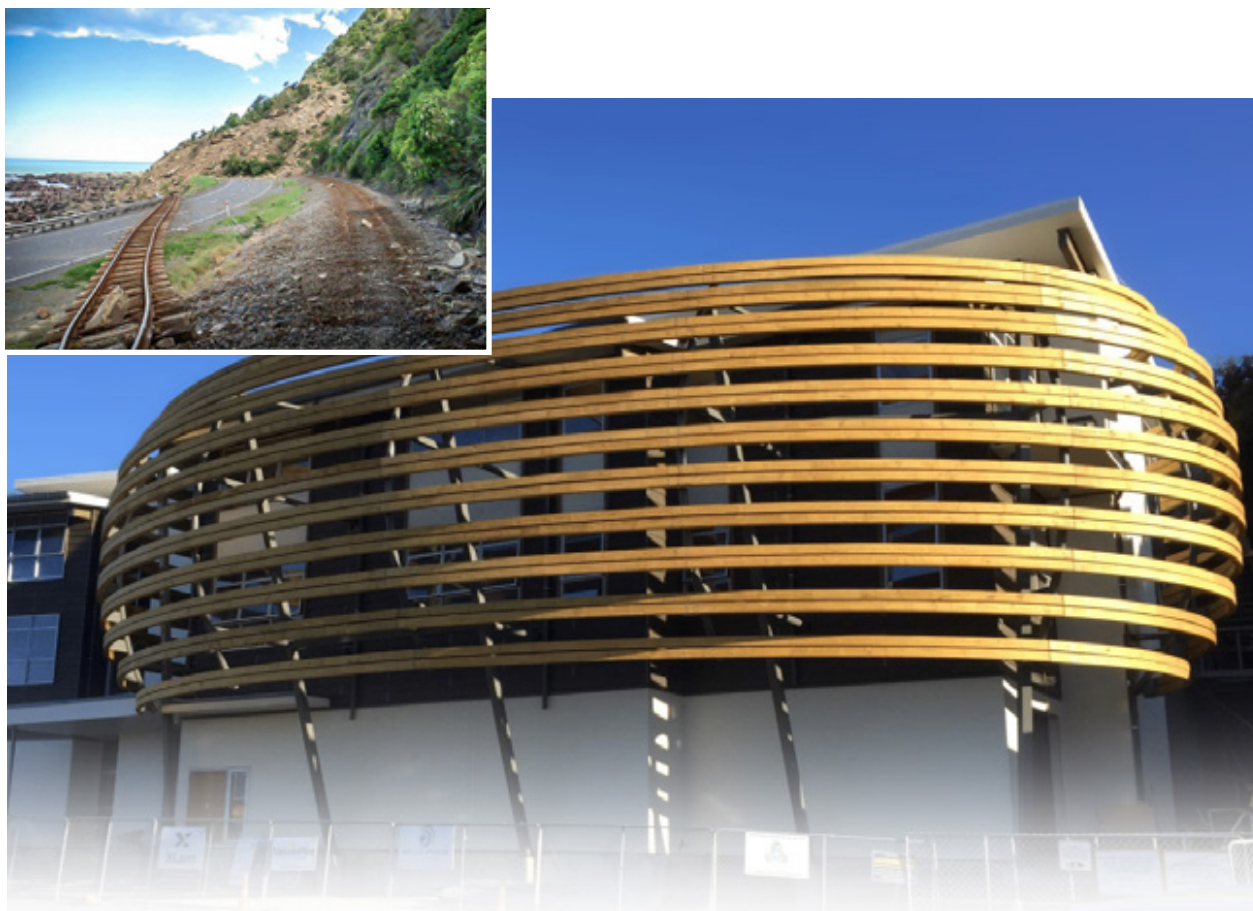
Figure 1: The multi-storey mass timber Kaikoura District Council building uses Pres-Lam technology as its lateral load resisting system. It was used as the base of operations following the magnitude 7.8 2016 Kaikoura earthquake.
