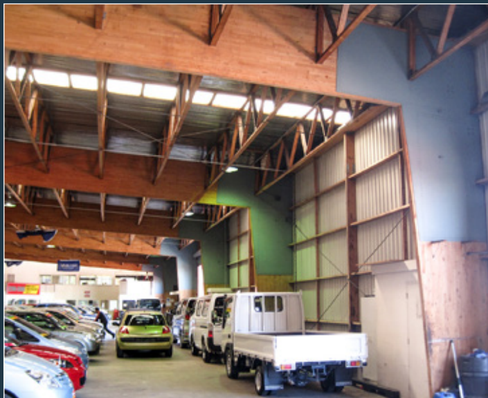
Timber portal frames for resisting lateral loads. Light steel wall and roof bracing. No damage in the 2011 Christchurch earthquakes.
