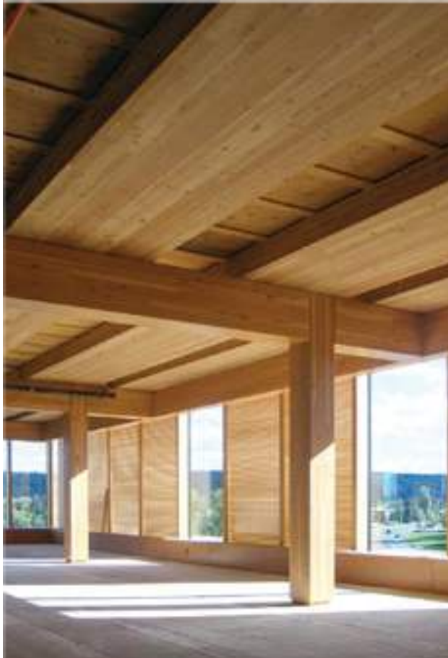
Gapped CLT Panels, Wood Innovation Design Centre, Prince George, Canada. Michael Green Architecture.
