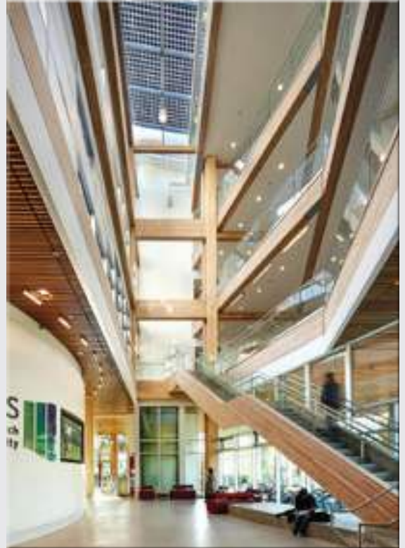
Post and Beam Atrium.
