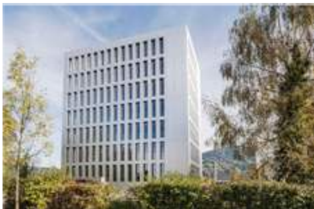
Life Cycle Tower One is an eight-storey office building in Dornbirn, Austria. The façade panels incorporated pre-fixed columns to improve installation time by reducing the number of lifts required.
