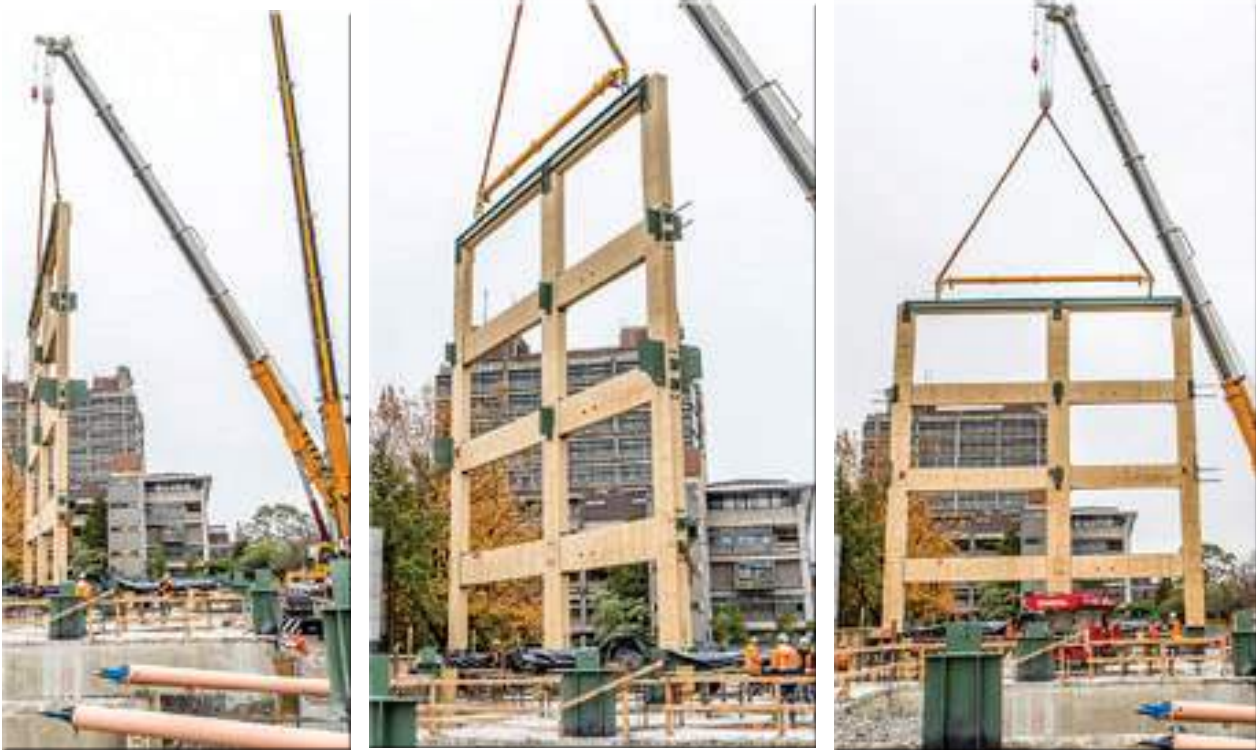
Moment Frames Lifted into Place – Beatrice Tinsley Building University of Canterbury.
