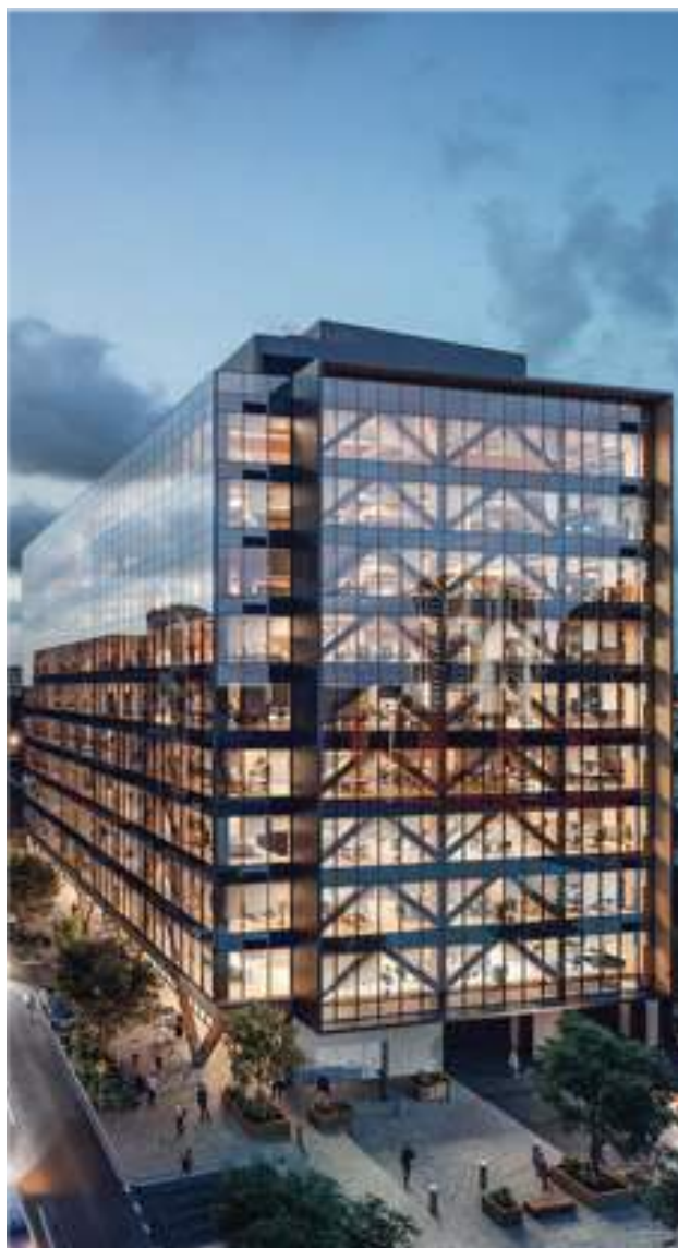
25 King Street, Brisbane: 10 storey post and beam structure.
