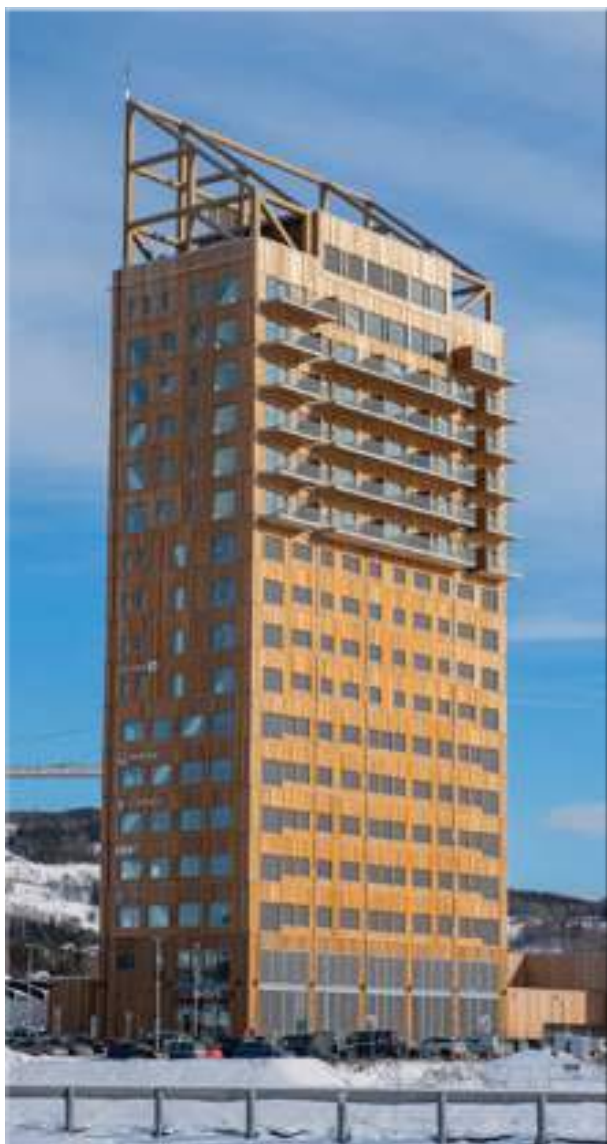
Mjøstårnet, Norway: 18 storey post and beam structure .
