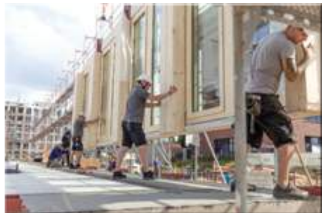
Life Cycle Tower One is an eight-storey office building in Dornbirn, Austria. The façade panels incorporated pre-fixed columns to improve installation time by reducing the number of lifts required.
