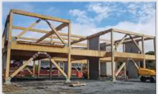
Hutt Valley Health Hub, Wellington. Timber chosen to facilitate a low damage design with high seismic performance, and to make the space feel welcoming.
